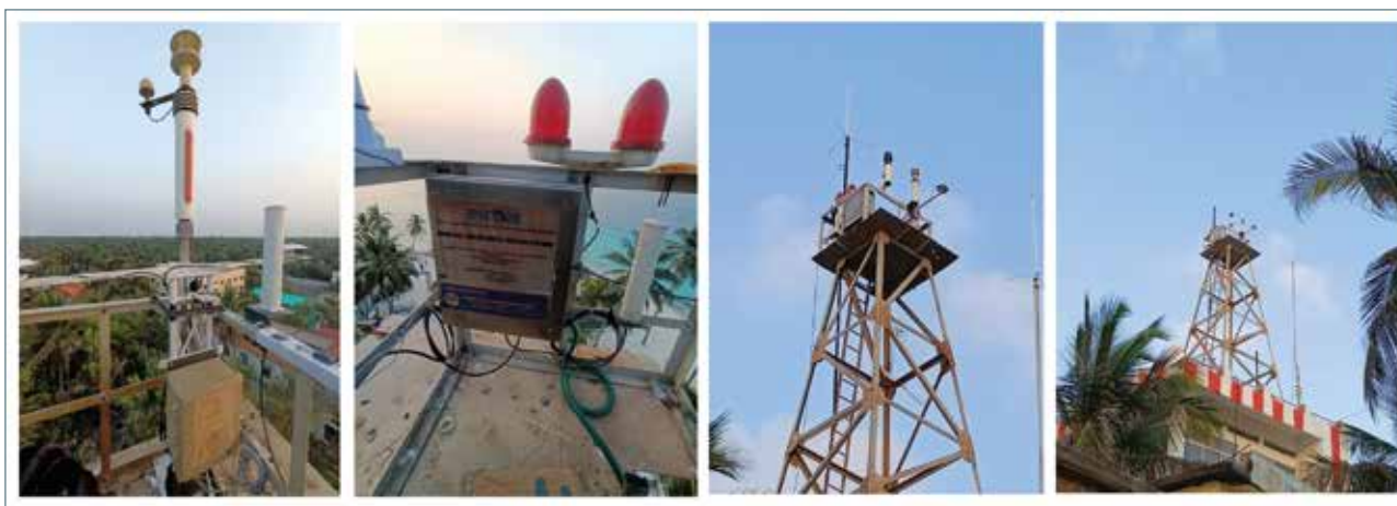
Fig. 6.9 Newly installed AWS in Port Control Tower, Kavaratti.
