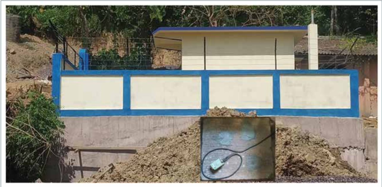
Fig. 6.21 The newly constructed GNSS and SMA recording room at Wandoor. The inset map at the bottom shows the SMA sensor.
