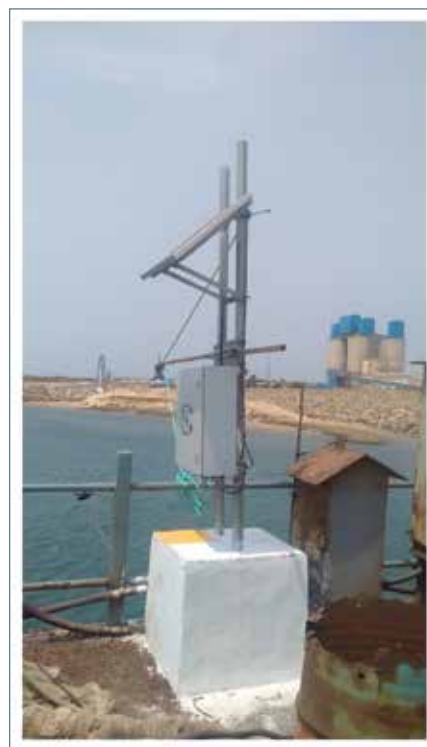
Fig. 6.13 Newly installed Radar Tide gauge system at Gopalpur port
