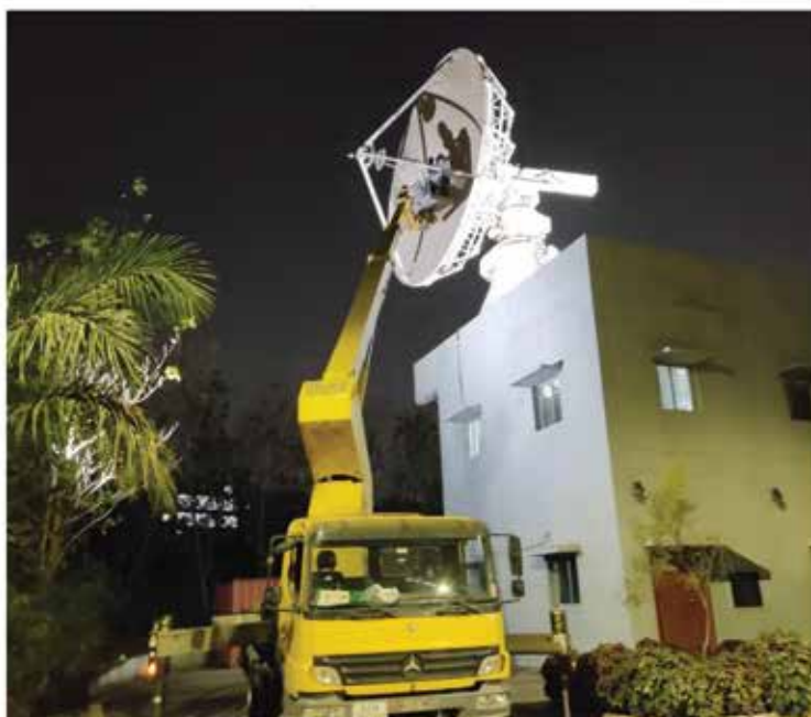
Installation, configuration & testing of the Noise cancellation filters at Oceansat ground station
