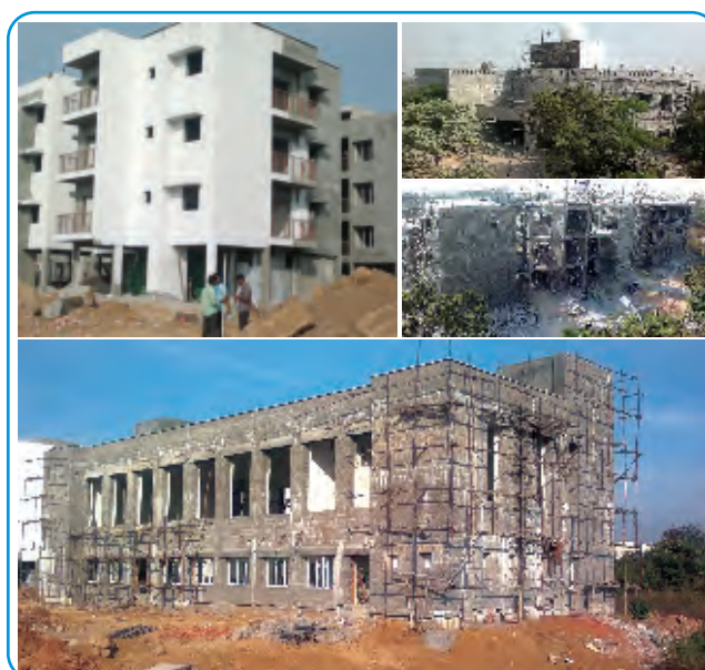
Figure 13.3: Expansion of ESSO-INCOIS building infrastructure in progress.
