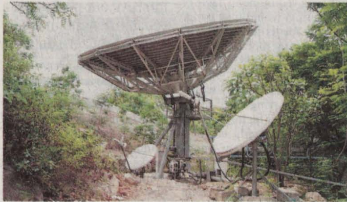
The VSAT hub antenna receives seismic/GPS data from remote field stations. — PHOTO: SPECIAL ARRANGEMENT
